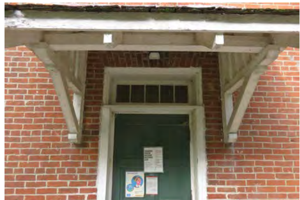
Door surround and transom at north entry on the east elevation.
