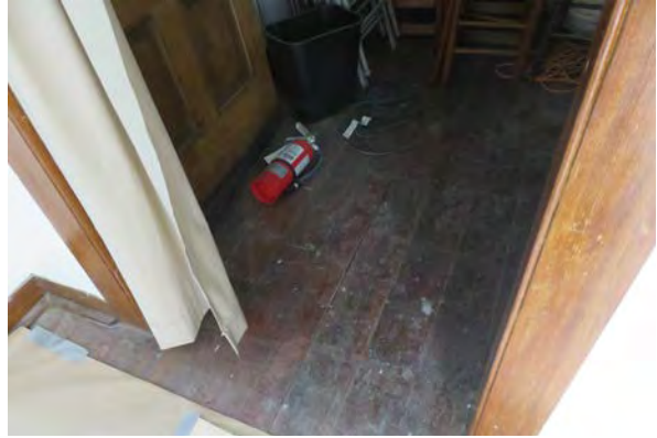
Typical wood floor at the second floor.
