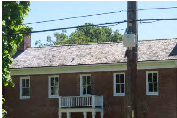
Roof at north elevation.
