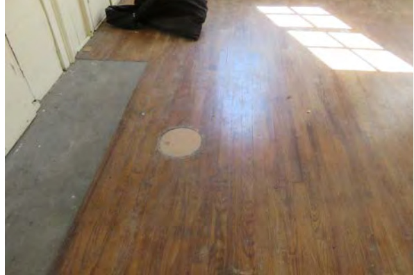
Repaired hole in the floor of the first floor east room.
