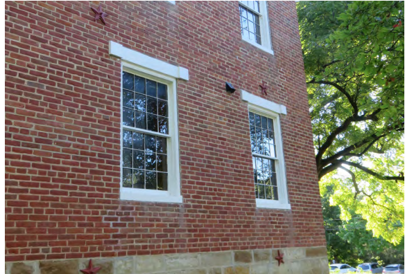
Sashes and surrounds that were repaired in 2016.
