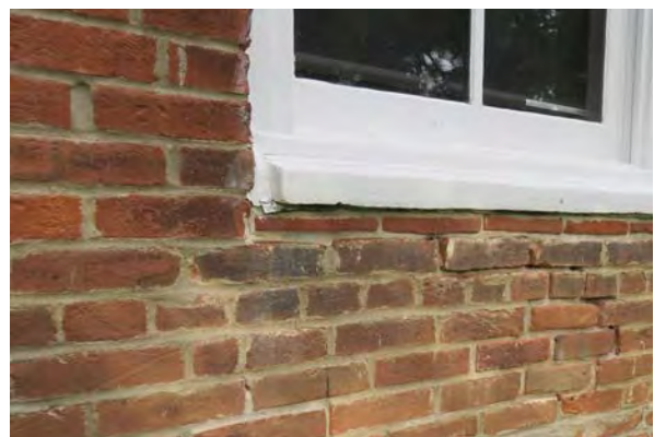
Sealant at window frame.
