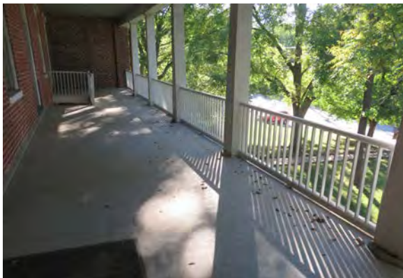
Second floor porch, looking east.
