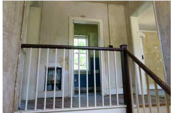
Landing at second floor
