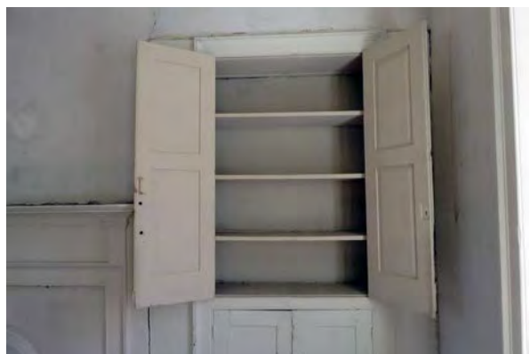
First floor east room built in, a defining feature.
