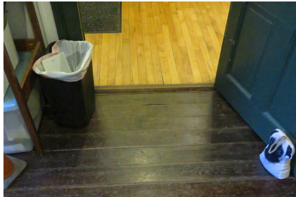
Transition between north foyer (above) and office (below) floors.
