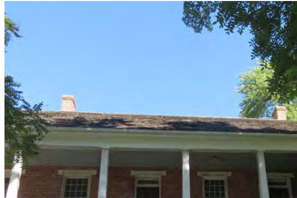
Roof looking south.
