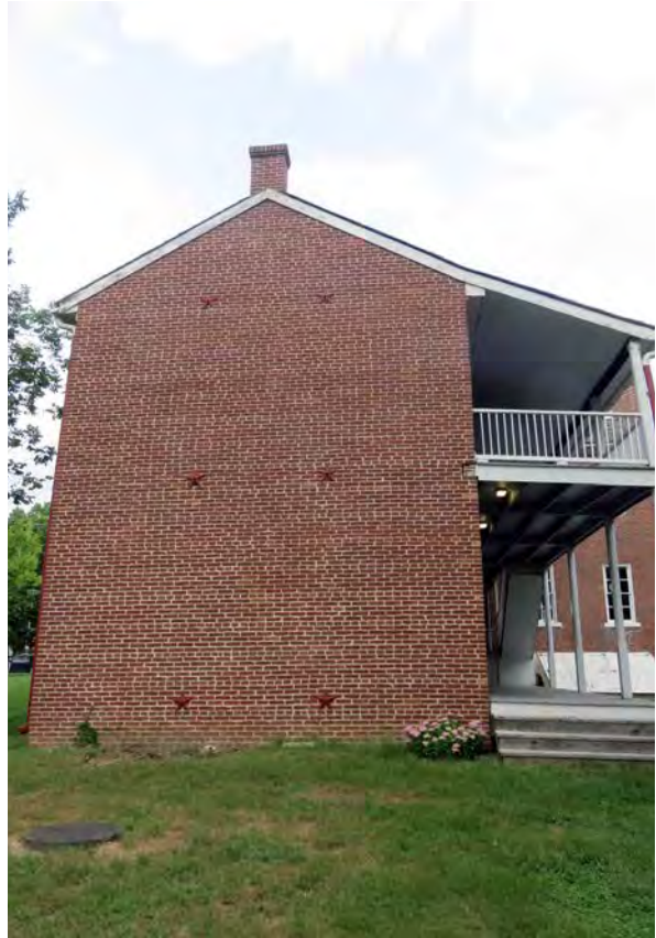
South elevation, rear addition
