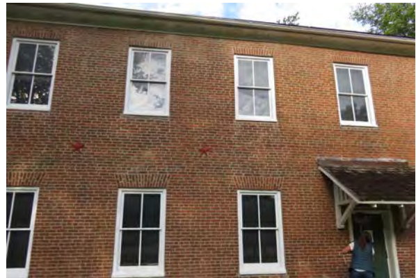
Exterior brickwork, with splayed lintels over windows.
