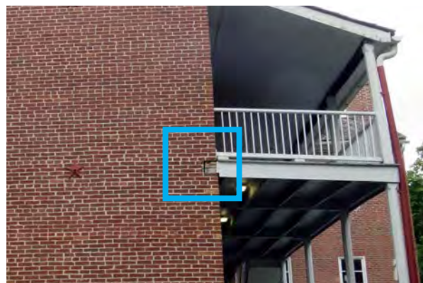
Exposed joist pocket, outlined in blue.
