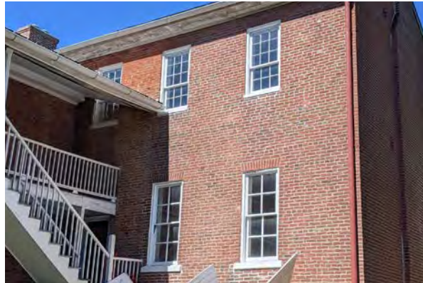
Window pattern on the rear of the original structure.
