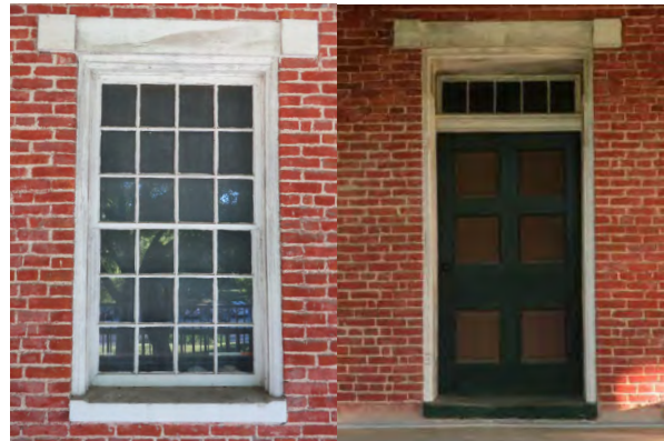
Doors and window as seen in 2021.
