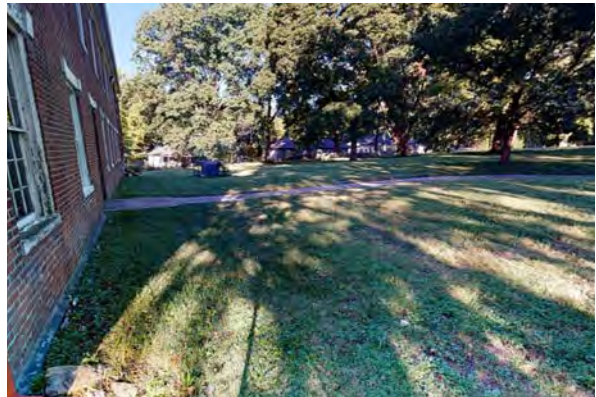
Path at the north elevation.
