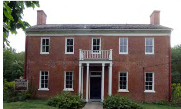
West Building, north elevation
