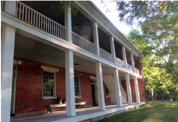
Porch and exterior stairs.
