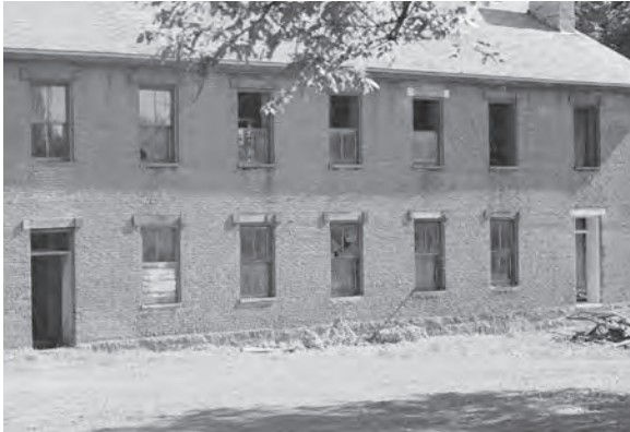
Detail of 1940s HABS photo showing two over two windows at the north elevation.
