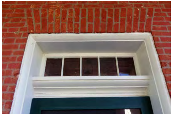
Splayed lintel at north elevation, a defining feature.
