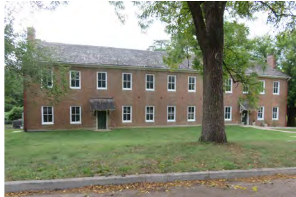
East Building, east elevation
