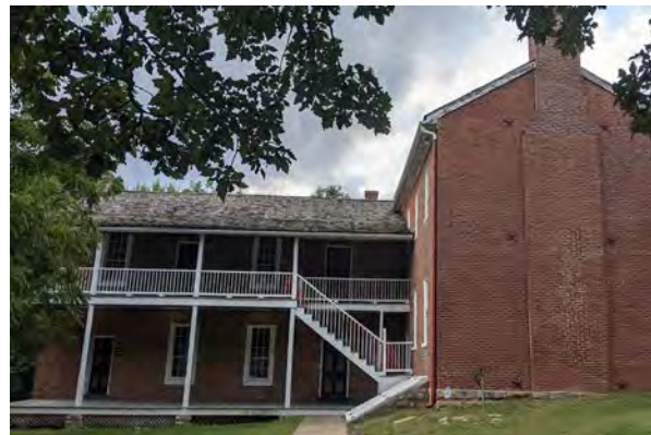
West Building, east elevation
