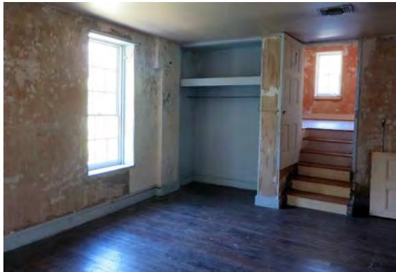
North bedroom in rear addition
