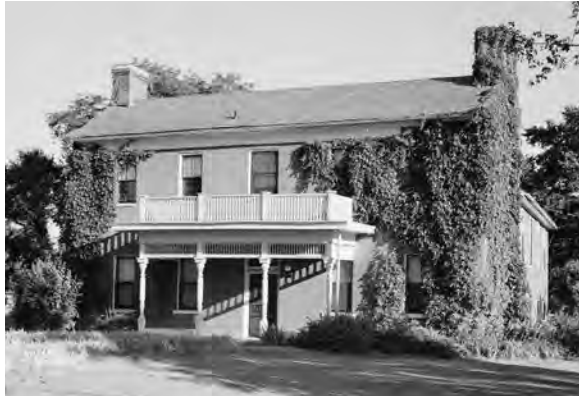
West Building, 1940, Photo courtesy of HABS KAN-3 by Lester Jones. [ https://www.loc.gov/item/ks0018/ ]
