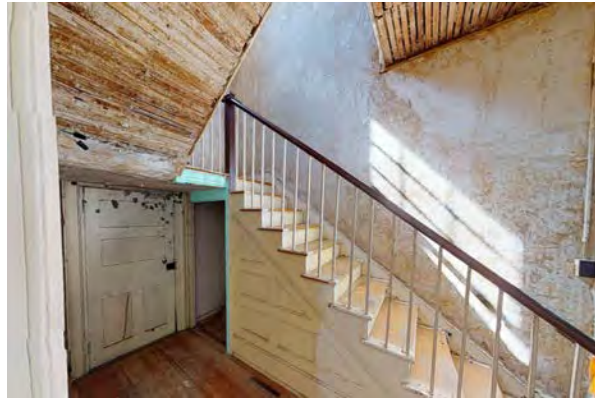
South door of foyer and stair, both defining features.
