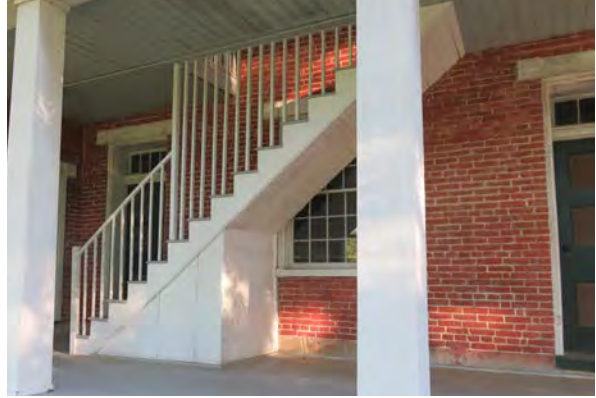
West staircase to the second floor of the porch. This is one of two potentially historic staircases at the porch.
