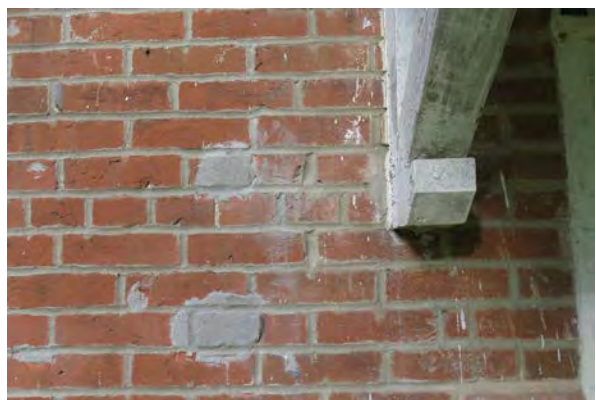
Patch executed in grey mortar.
