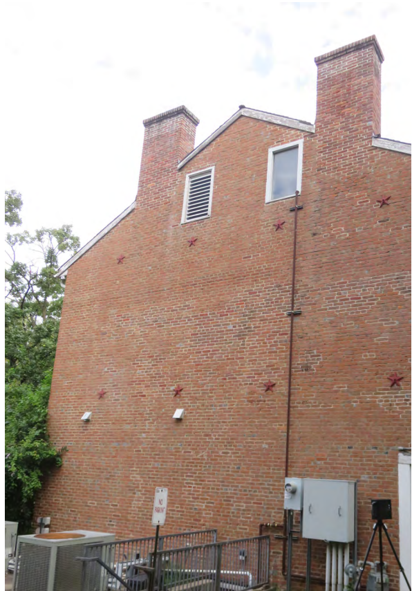
East Building, south elevation
