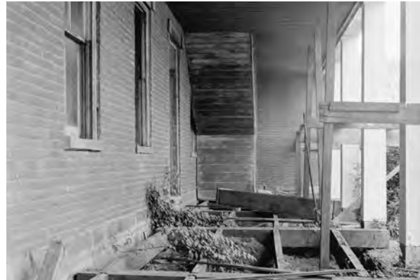
1940s HABS photo showing missing porch floor at the first floor. Note that the staircases is still intact and may be original.
