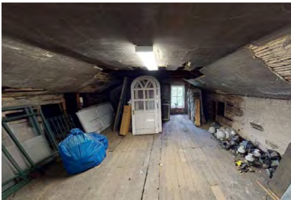
Attic, looking north.
