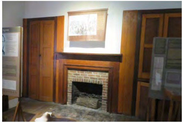
Built-ins in second floor southwest room.
