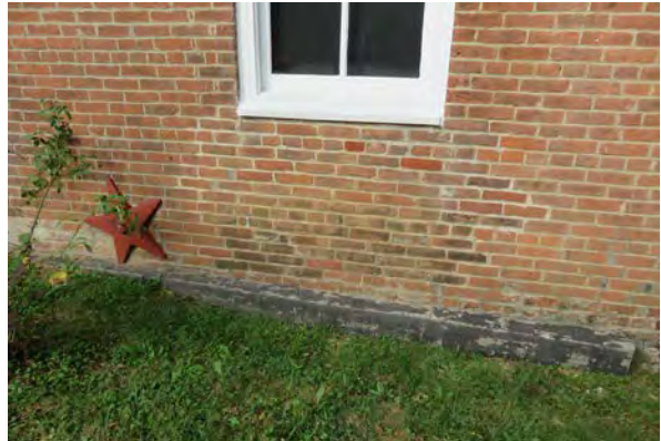
Area of repointing and brick replacement at the east elevation.
