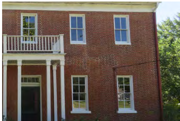
Window pattern at the north elevation.
