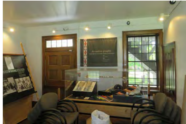
Exhibit room between small exhibit space and west foyer. This area is used to store materials from the west room which is under repair.
