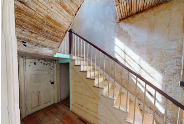
West Building. South door of foyer and stair, both defining features.
