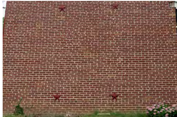
Common bond at south elevation.
