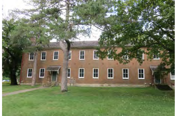
East Building, west elevation.
