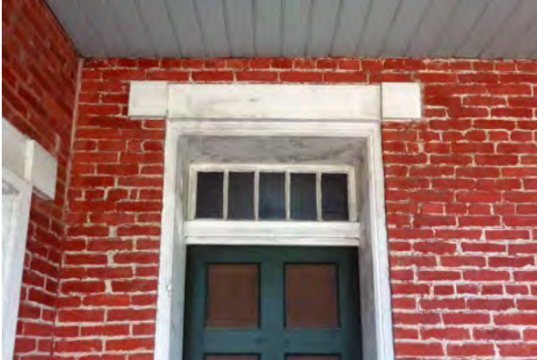
Transom and lintel with wood blocks.
