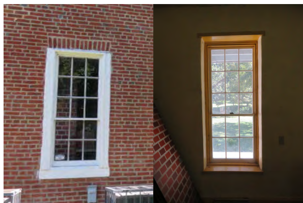
Nine over six double hung window, exterior and interior from the rear addition.
