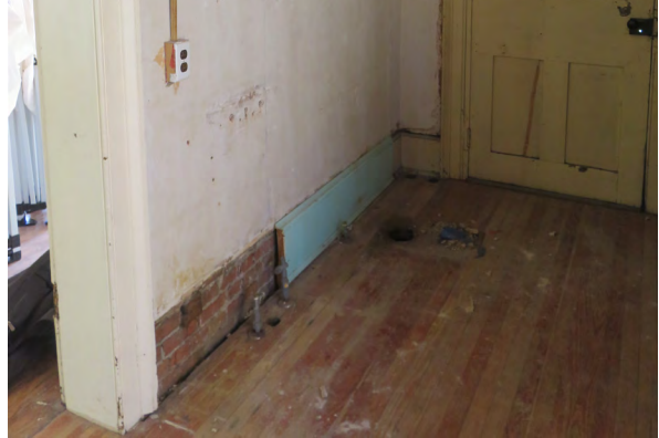
Exposed portion of brick wall below plaster in foyer.
